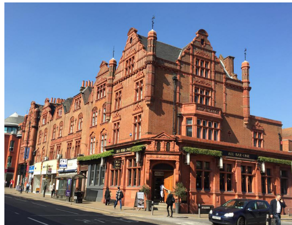
28 Bank Buildings, Wimbledon Hill Road
